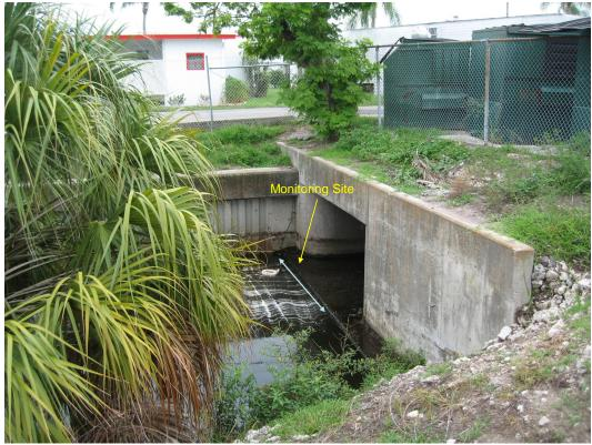
b. Box Culvert Discharge Monitoring Site
